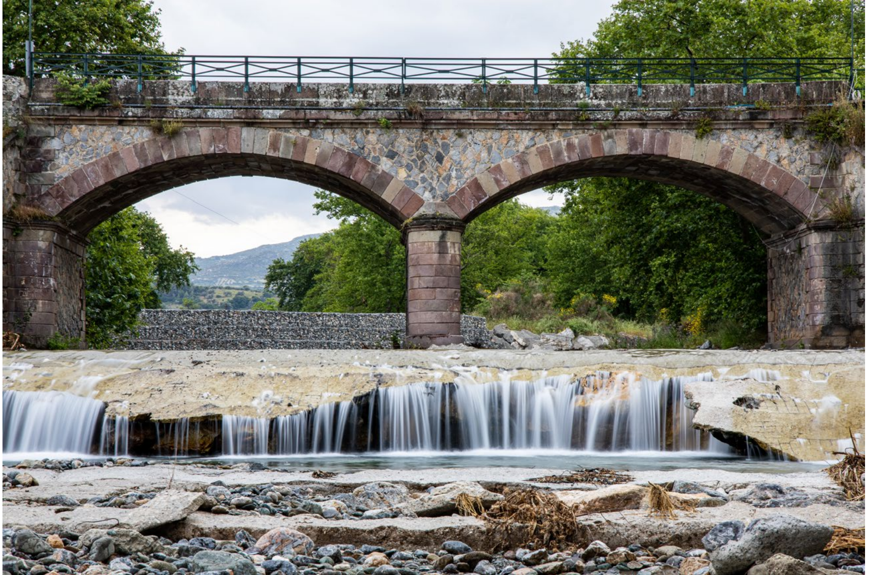
The bridge of Monodri
