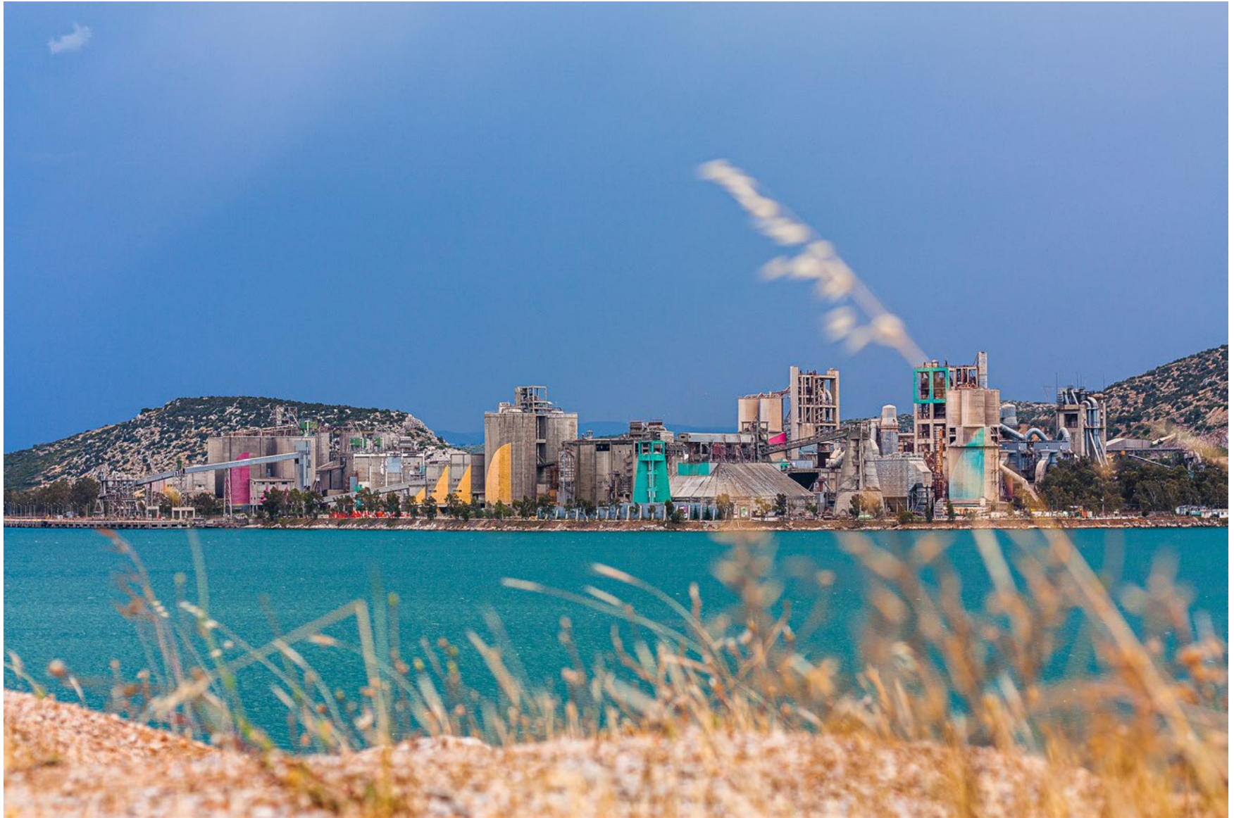
The old cement factory of Chalkis
